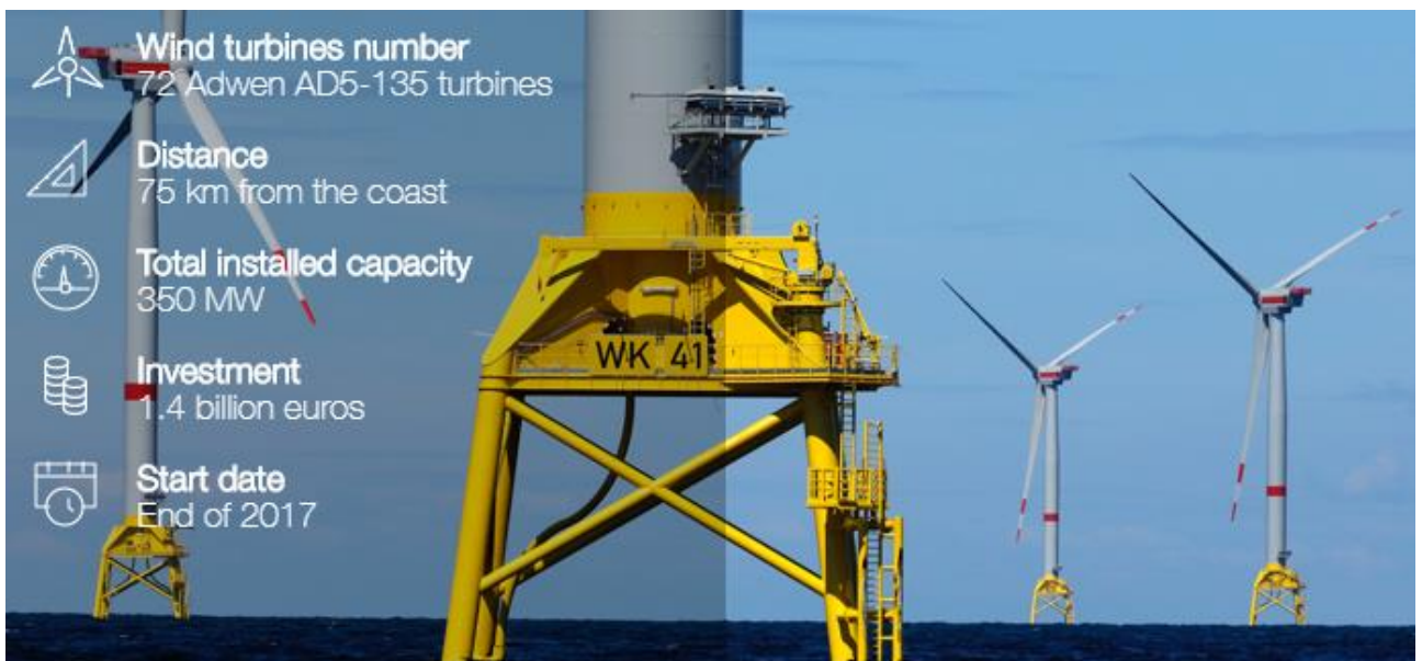
Figure 12. Wikingier offshore wind farm (IBERDROLA) was inaugurated in October 2018. 280 piles were driven into the sea bed to hold the foundations. Measuring 40 metres in length by 2.5 metres in diameter, and a unit weight of 150 tonnes, they were all built by Spanish company Windar.
