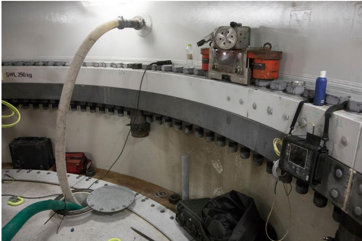
Figure 12: Bolting and grouting in progress, source: Boskalis 1 .
