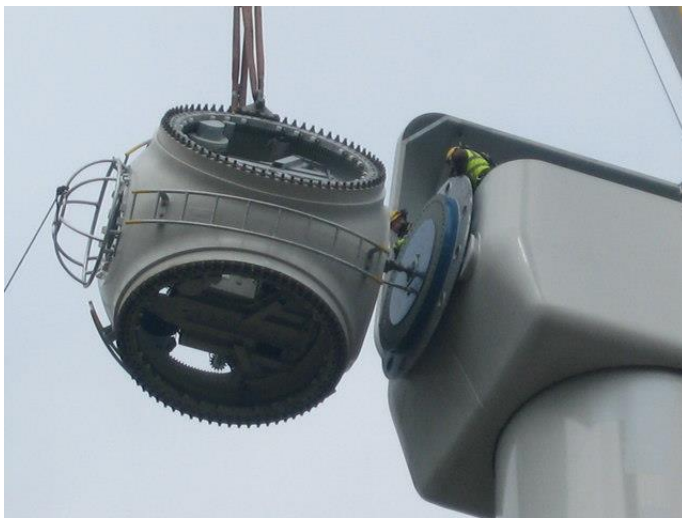
Figure 2: Wind turbine hub being installed. 1
