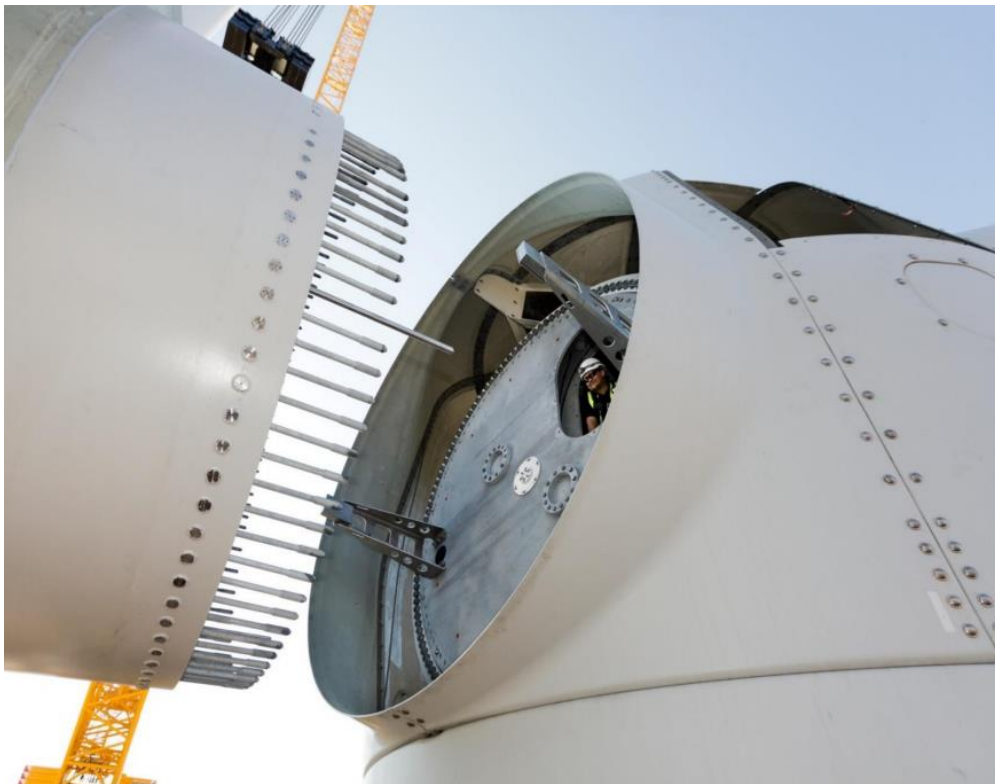
Figure 16: Image of a blade being connected to its hub. The T-bolt principle is used. The barrel nuts can clearly be seen around the circumference of the blade root. 1
